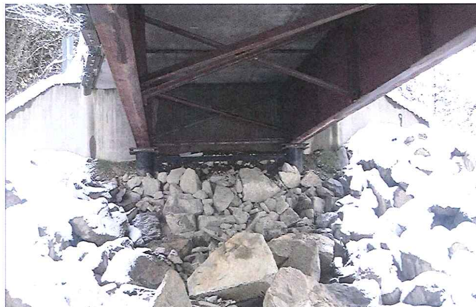
CK2444 Abutment Left Bank
