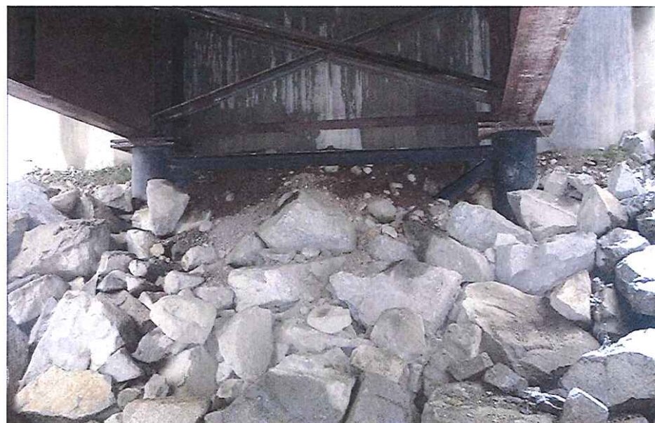
CK2444 Abutment Right Bank
