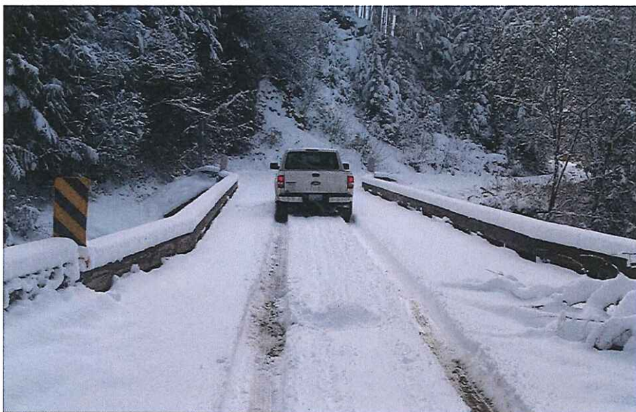
CK2444 Approach Right Bank
